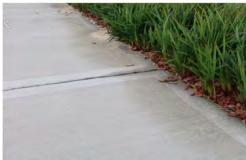
Broom finish concrete path with trowelled border
