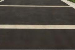
Asphalt driveway with 500mm wide acid etched plain concrete bands
